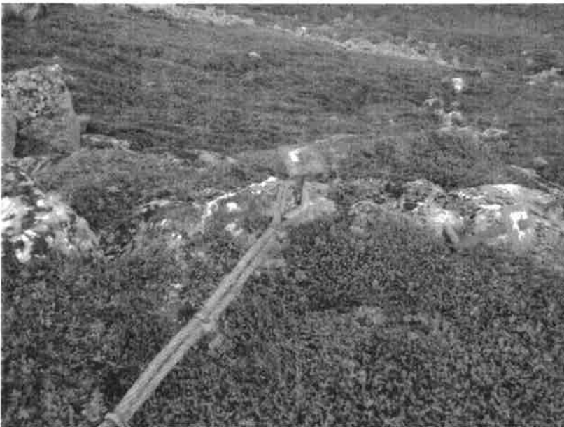
Figur 14. Festemetode for sikringswirer
